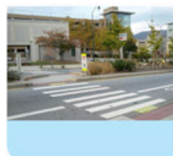
Marked crossings and pedestrian refuges
