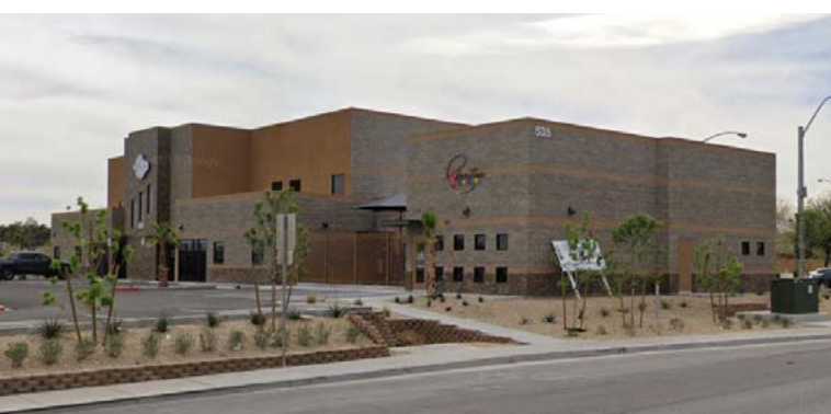
Top: North Las Vegas City Hall sits just outside site A. Middle: Rendering of mixed use, retail development in the Lake Mead Village West district. By Bunnyfish Studios. Bottom: New Expertise Barber and Cosmetology Institute on Lake Mead Blvd, near site D.
