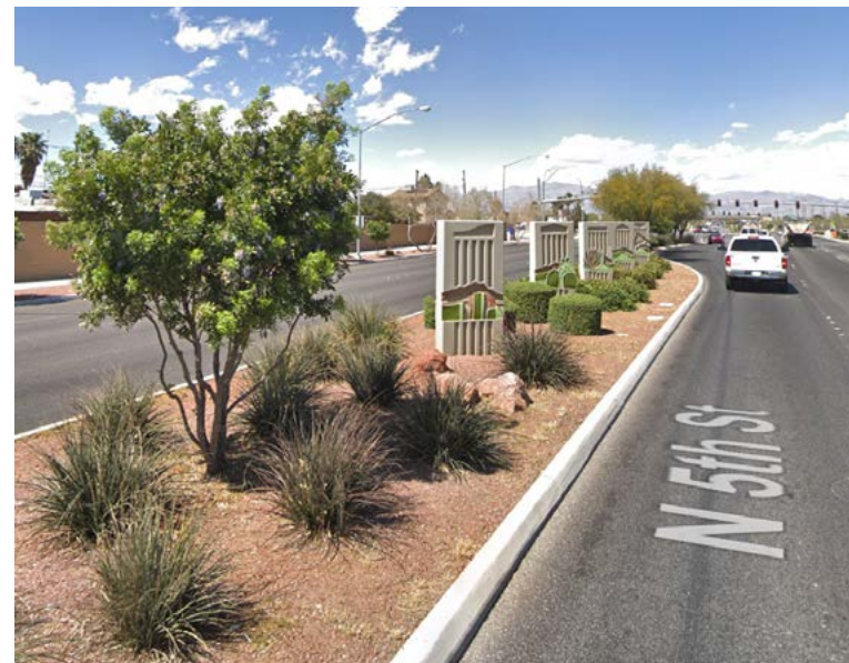
Photo of North Fifth Street improvements.
